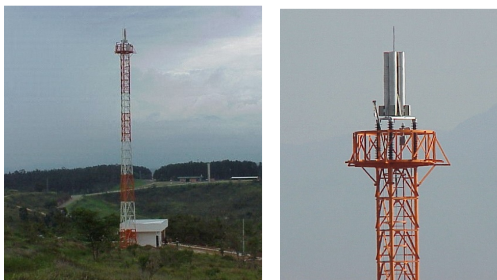
Figure I.1 – General view of the RBS and detail of the rocket platform on the tower top
