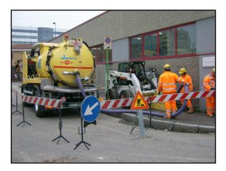
Figure I.1 – Trench saw combined with suction machine
