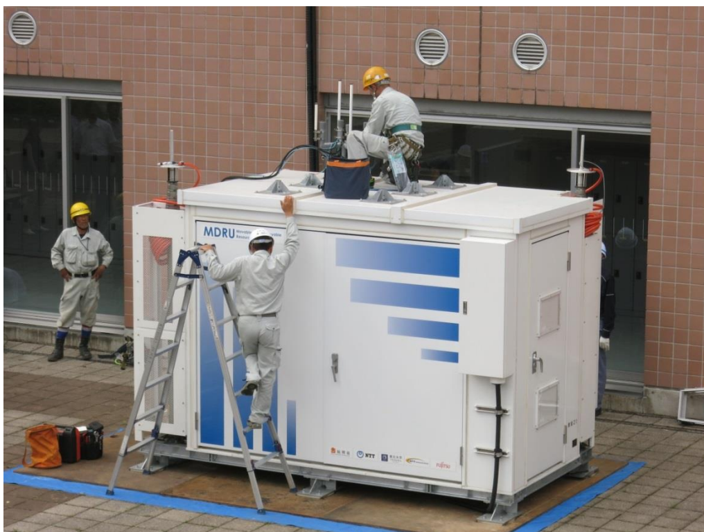
Figure I.3 – Deploying and configuring a movable and deployable ICT resource unit at a remote site
