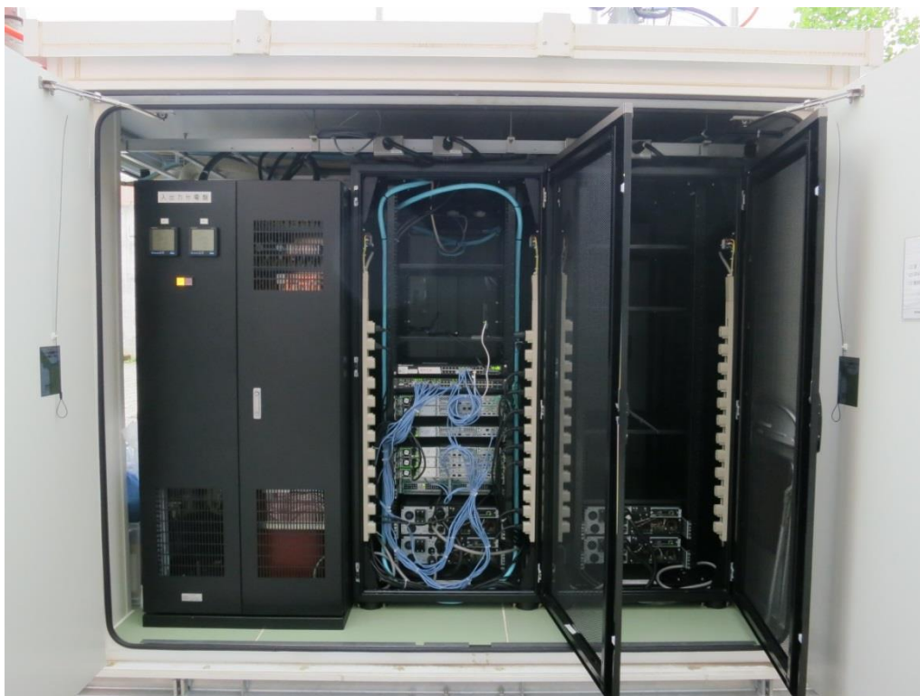
Figure I.6 – Components inside a movable and deployable ICT resource unit
