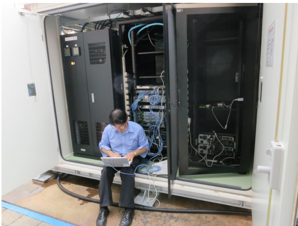
Figure I.5 – System configuration and start-up of a movable and deployable ICT resource unit
