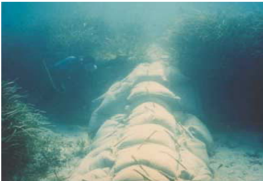
Figure I.2/L.28 – Protection performed by positioning sand-cement bags under, laterally and above the cable
