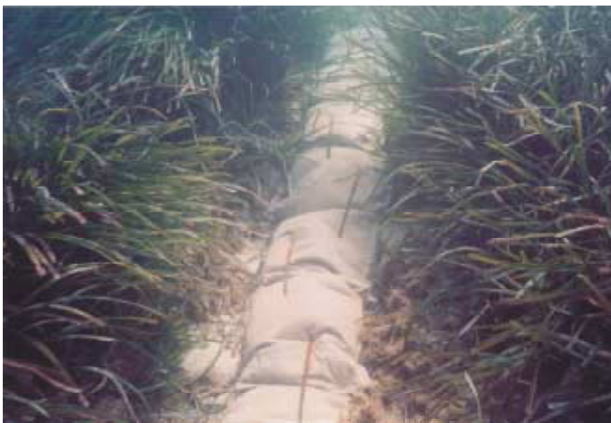
Figure I.4/L.28 – Photo of an example of external cable protection using cast-iron shells and additional sand concrete bags
