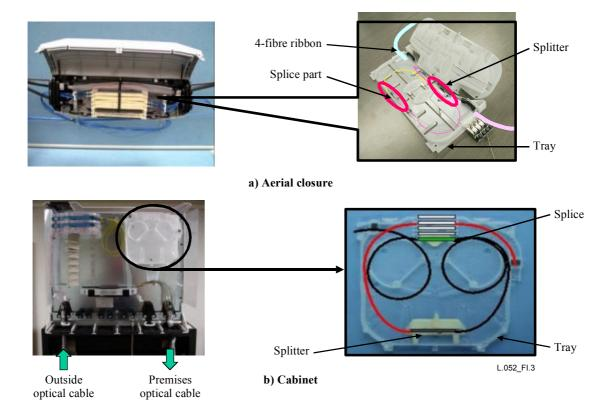
Figure I.3/L.52 – Photograph of a (fibre optic) branching component accommodated in an optical closure and a cabinet
