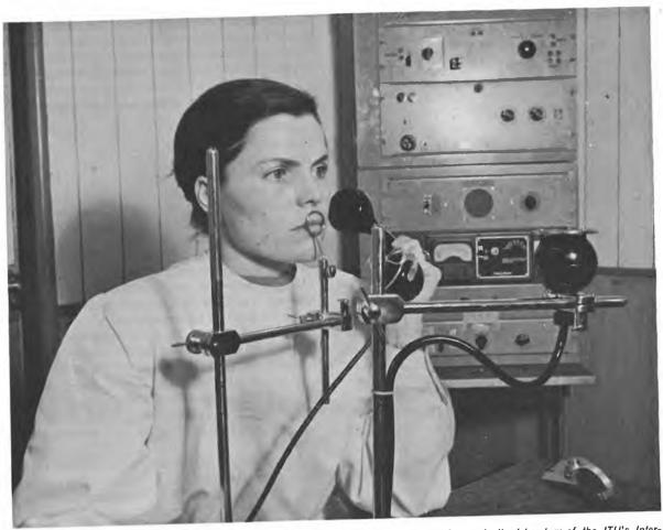
Mademoiselle Ursula Landvogt, one of the operators in the CCITT laboratory of the ITU, making speech tests.
